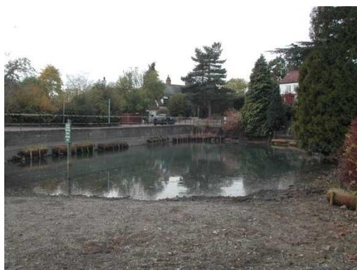
**Refilling:** the large pond was filled from a stand pipe under licence from Three Valleys Water. The small pond was allowed to fill naturally from rain water and was full by mid-November 2003.
